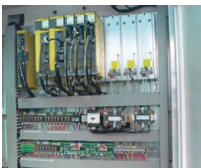
C.E type electrical components easy maintain and after-service job.
